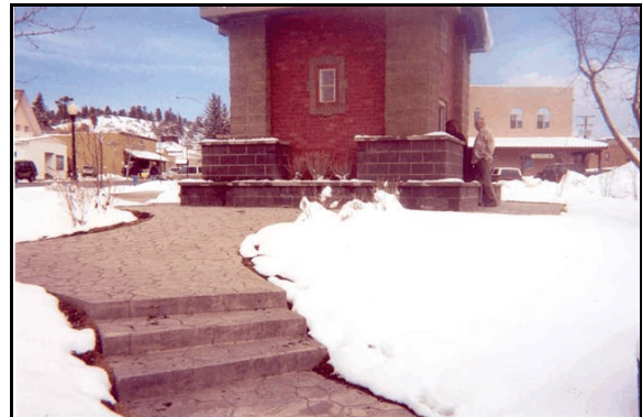
Water from the Great Pagosa Hot Springs heats several customers in the Town of Pagosa Springs including the town square. (Photo: Governor’s Office of Energy Management and Conservation)
